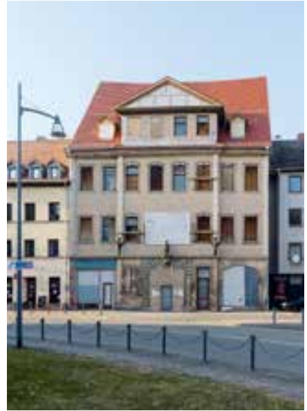
Weissenfels, emergency repairs to the empty Court Marshal's House, 2018
